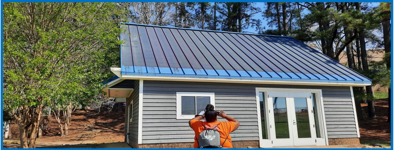
The student's workshop was held in the Solar garage.
